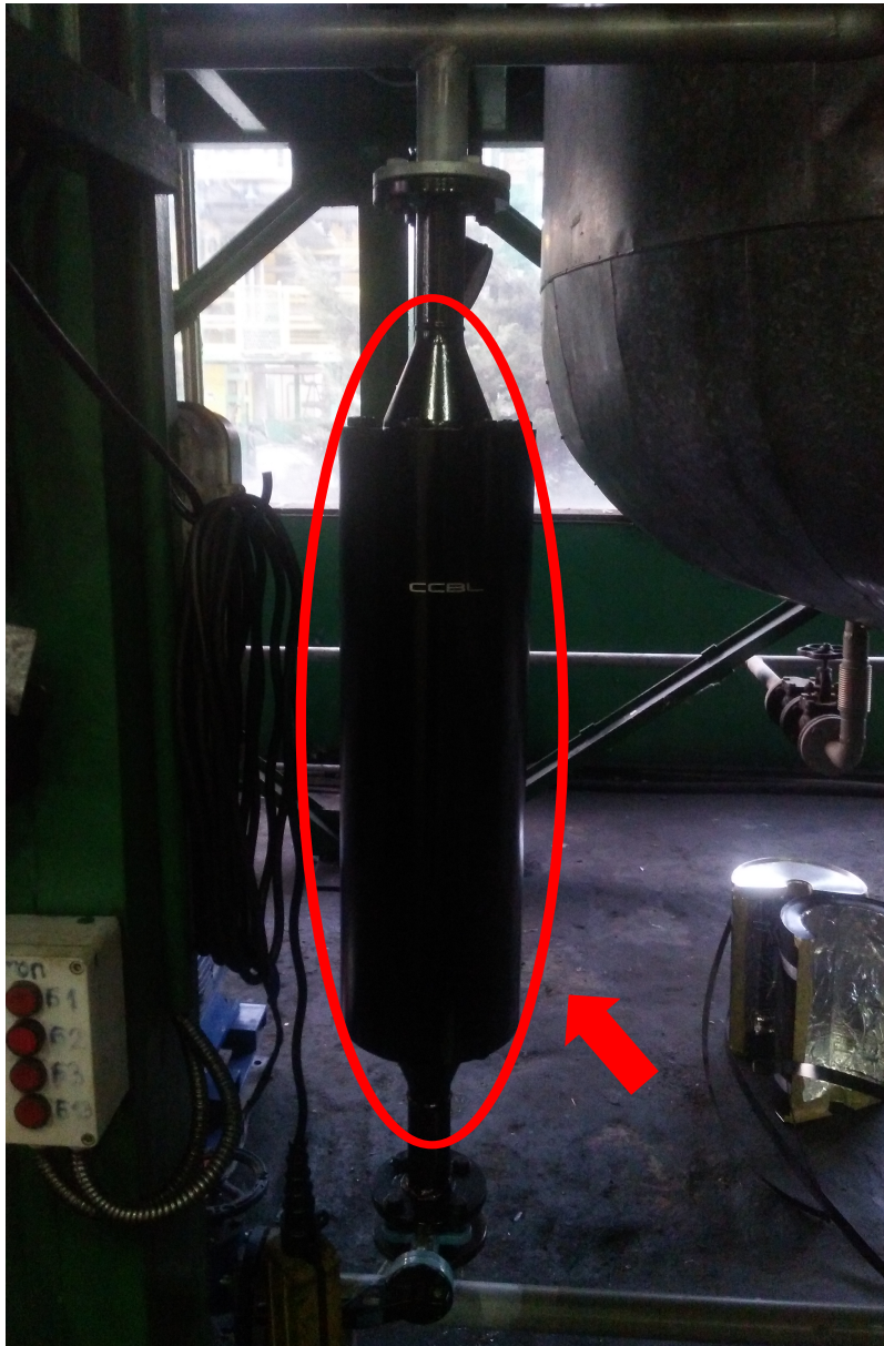
PRISTA OIL Blending Plant at Ruse (Bulgaria). The 10 cubic metric tank with integrated CCBL® JET unit.
